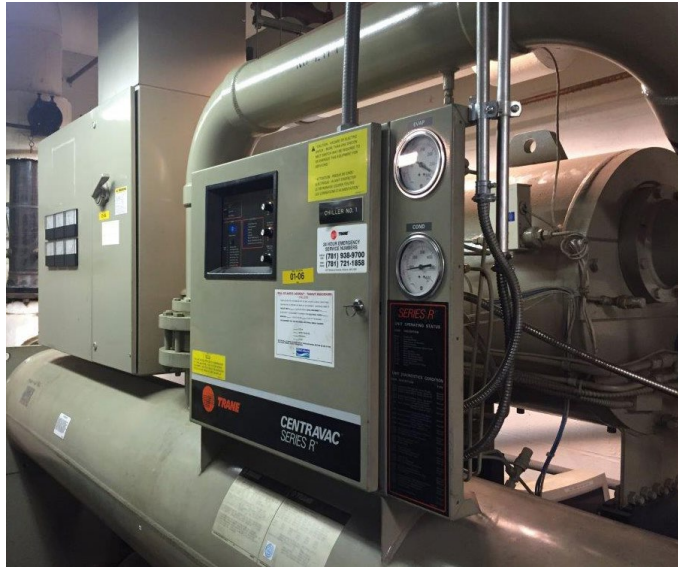
Prior to Upgrade - old controls
